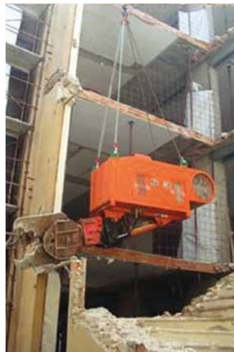
A.D.M. – Aerial Demolition Machine
